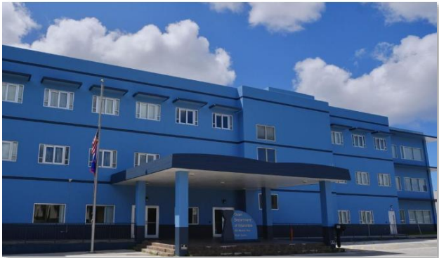
Figure 1: GDOE Central Office, Tiyan, Guam
